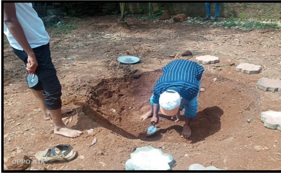
Digging for the Pond
