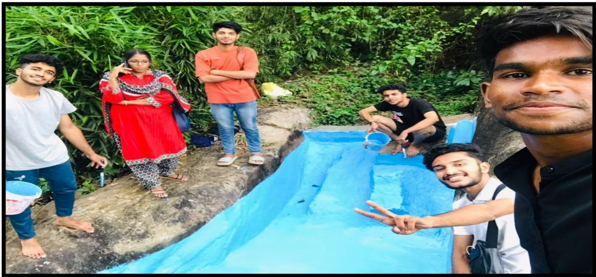
Painting Works for Make the Pond Water Proof
