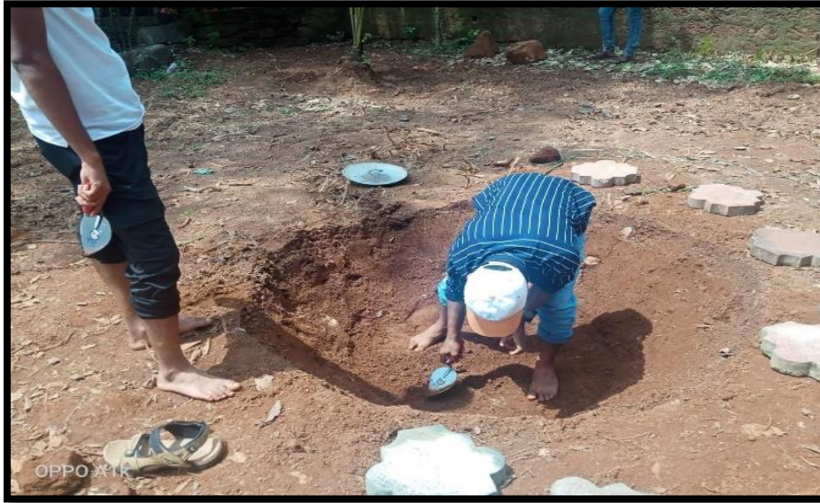
Digging for the Pond
