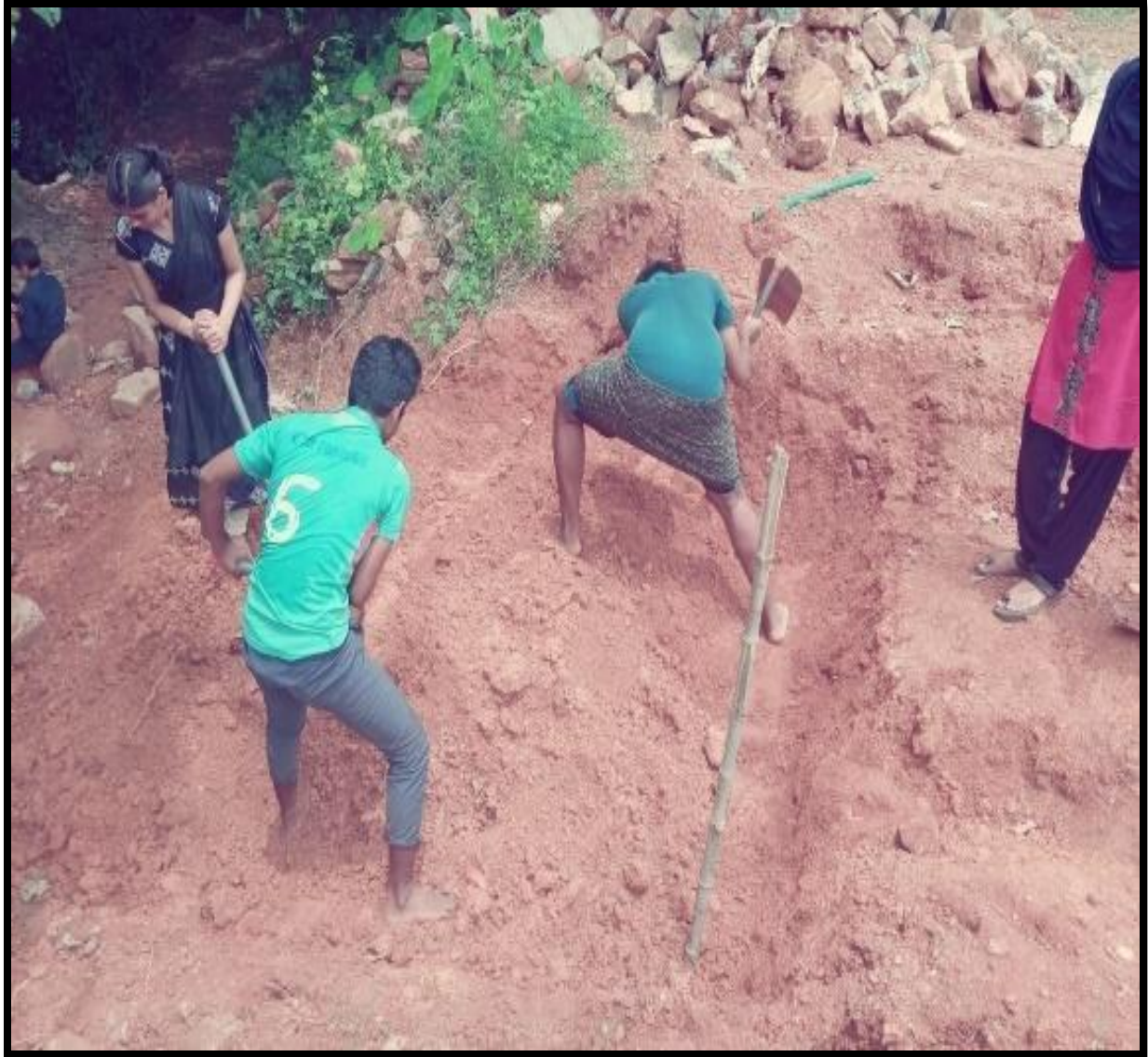
Constructing Rain Water harvesting Pit with the help of NSS volunteers
