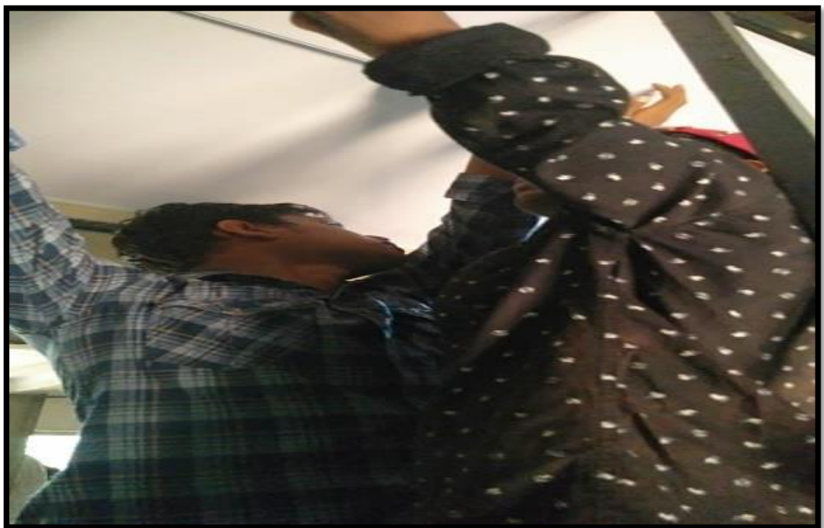
Fixing the Ceiling in Appu's house
