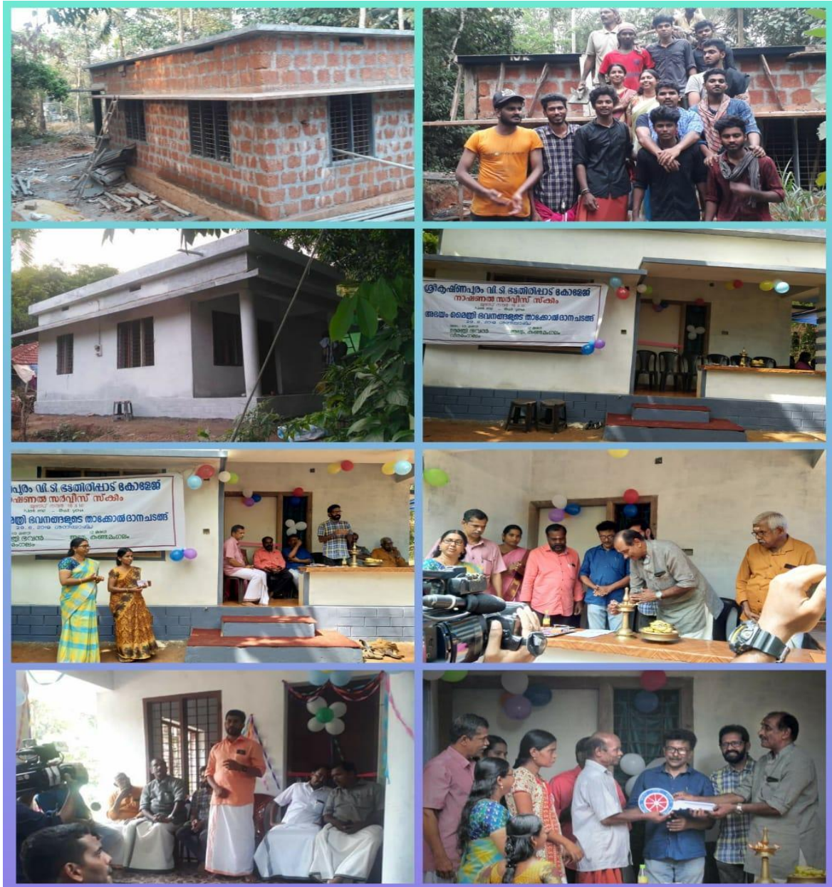
Completing the Home construction and Key hand over
